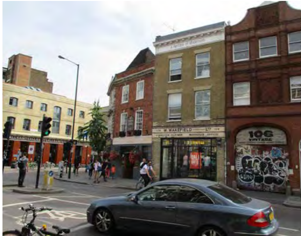
106 Commercial Street - Main Entrance with Grafitti covered shutters
