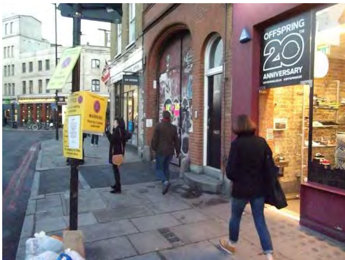
Figure 1: View north along Commercial Street with site entrance on right (brick archway)
