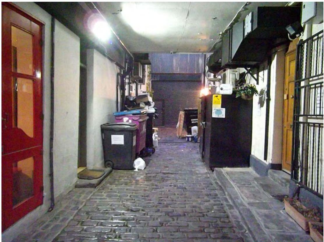
Figure 3: Service entrance on Hanbury Street
