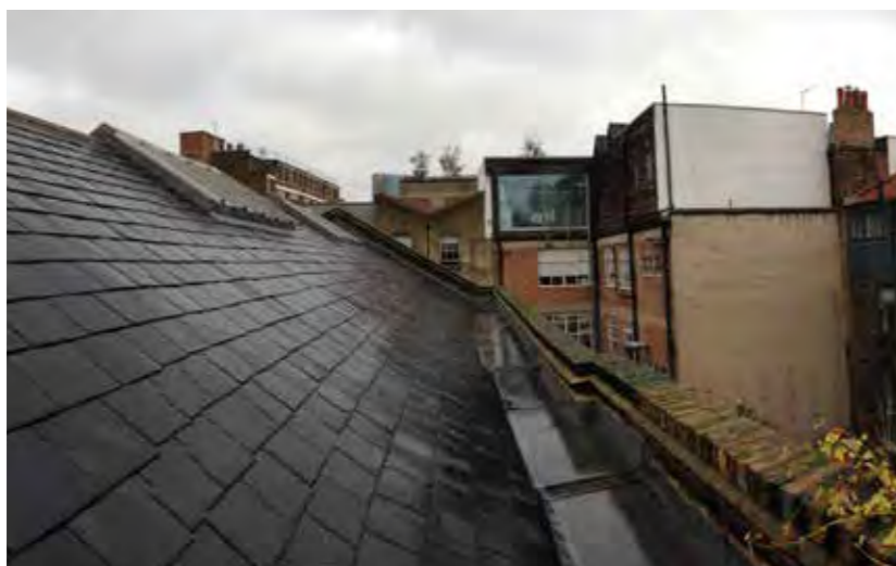
Image 03: east parapet, looking north.
