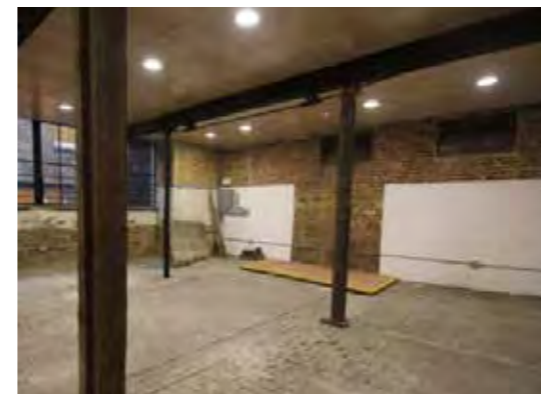
Figure 6.1 – Unusual propping to first floor east wing
