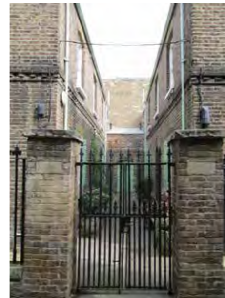
Existing Puma Court View
