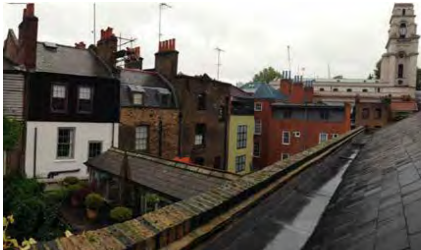
Image 02: east parapet, looking south.
