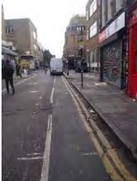
Figure 3.16 Hanbury Street double yellow lines and parking bays
