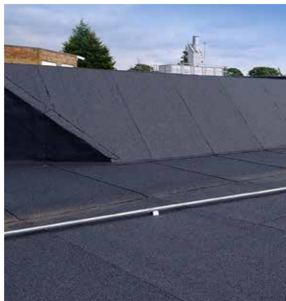
03. Bituminous Roof Membrane
