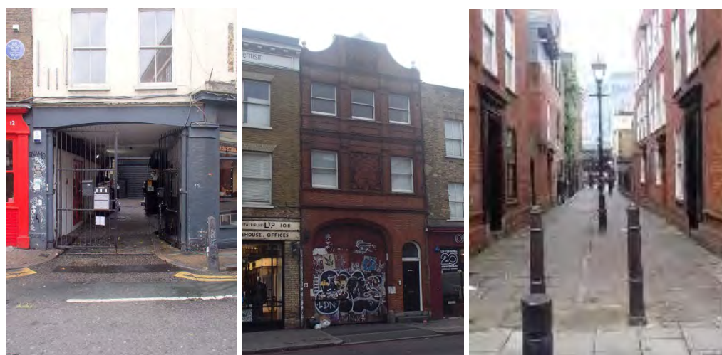
Figure 3.3 Accesses to 106 Commercial Street from Hanbury Street (left) Commercial Street (middle) and Puma Court (right)
