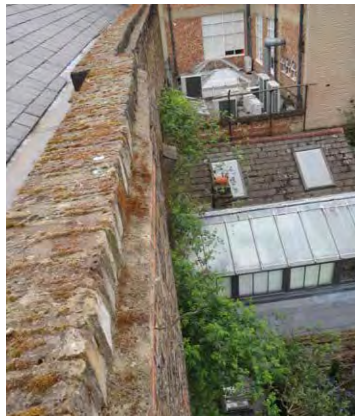
Image 05: east parapet, looking north.
